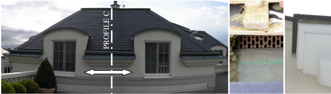
FIG. 10: a: General View Tested Eaves; b: Outside Horizontal Cross Section Eaves; c: Open Seam Sheeting
